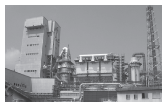
DOWA Group Recycling Plant
